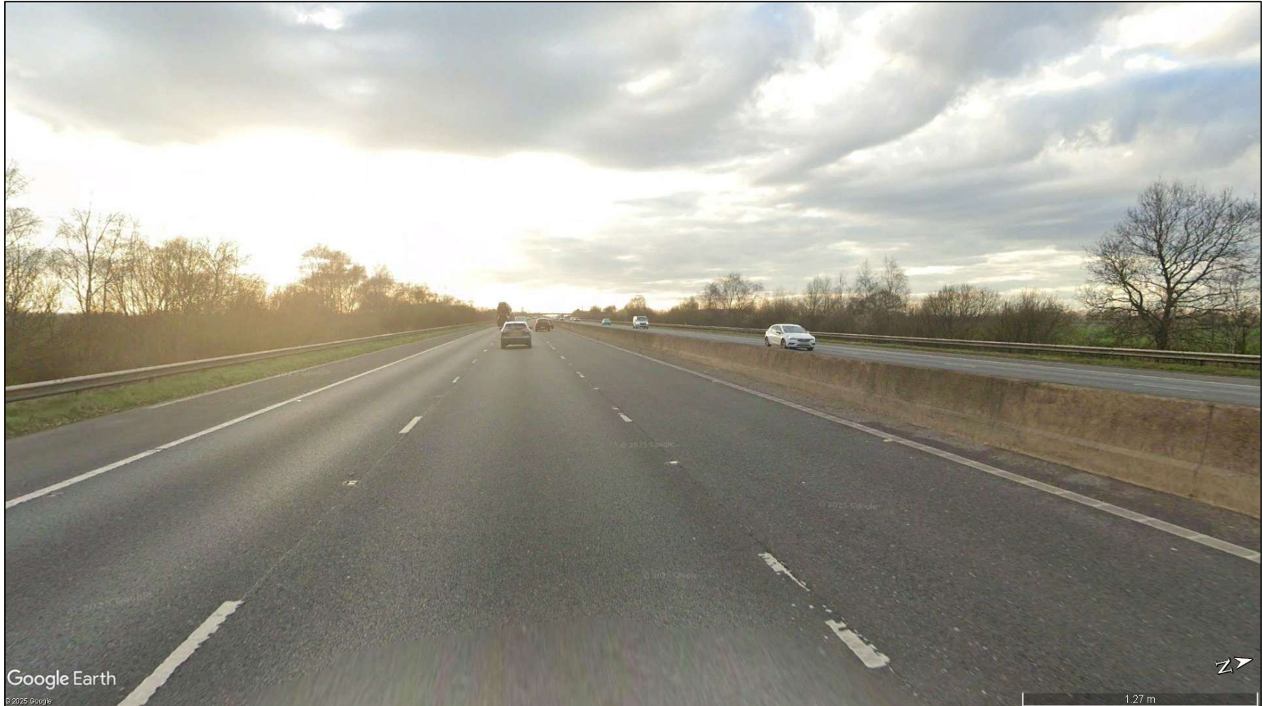
Significant roadside terrain and vegetation screening at road receptor A63 (road user travelling west)
