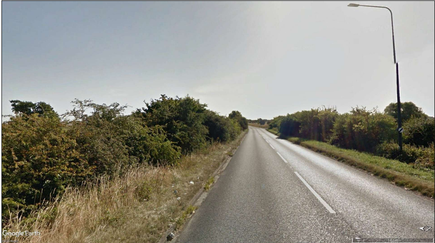
Significant roadside vegetation screening at road receptor D1 (road user travelling east)
